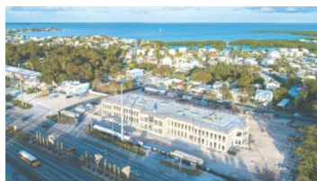
COLLEGE CONSTRUCTION PROGRESSES WITH FALL OPENING NOT FAR OFF March 23, 2021
